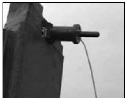
9. Fully released shackle ready to be removed from component.
